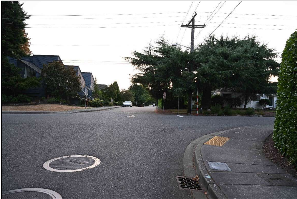
Figure 1 - West Bound on NE 5 th (Note no street lights on corner)
